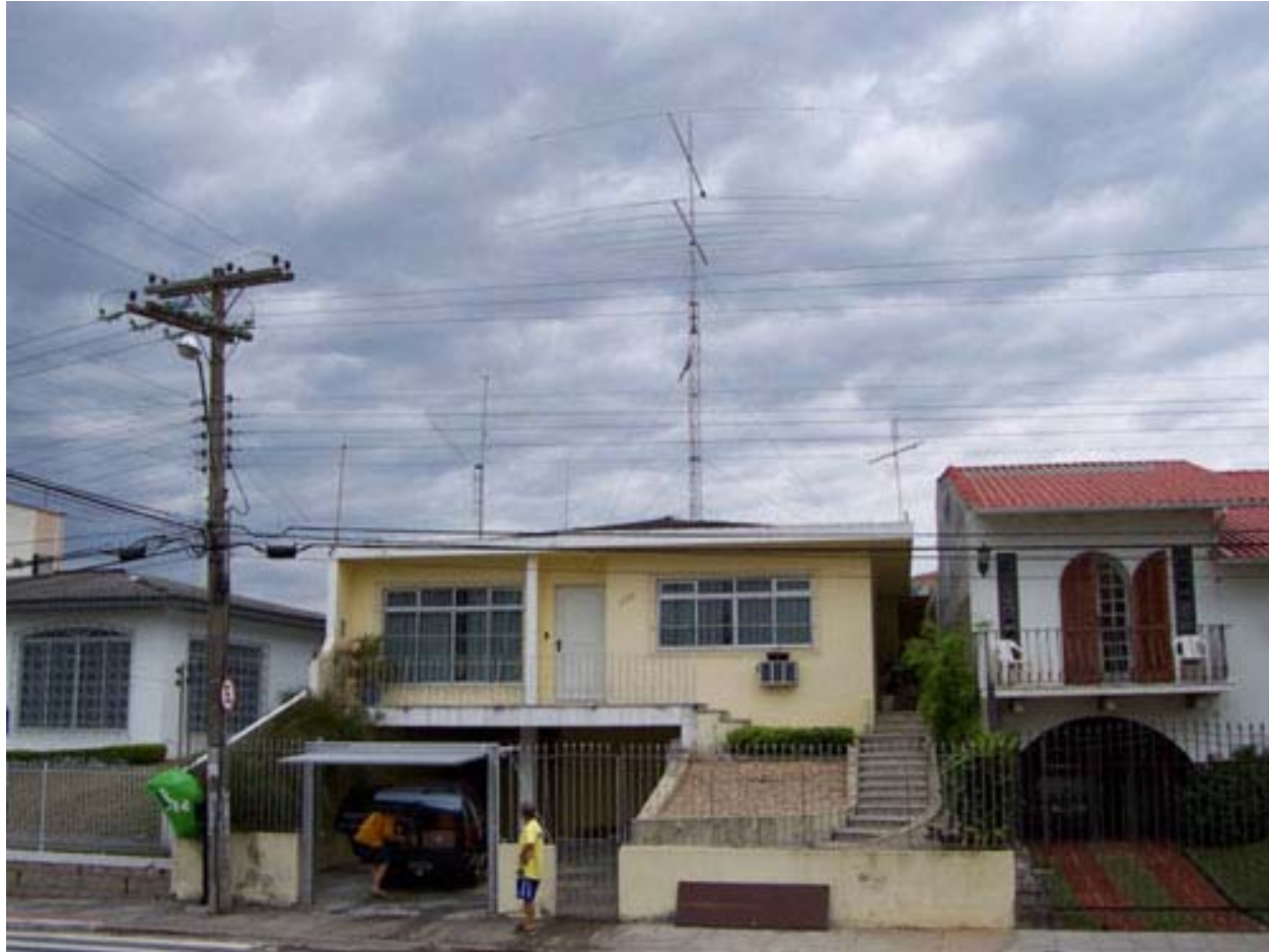
Antenna installation: PW4X. 50-foot tower, log-tribander and 2-ele. 40 ( UT4UZ )
