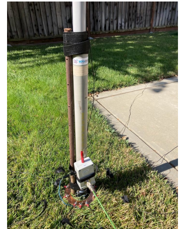
Figure 1. Base of the antenna showing the mast, radial connections, and matchbox
