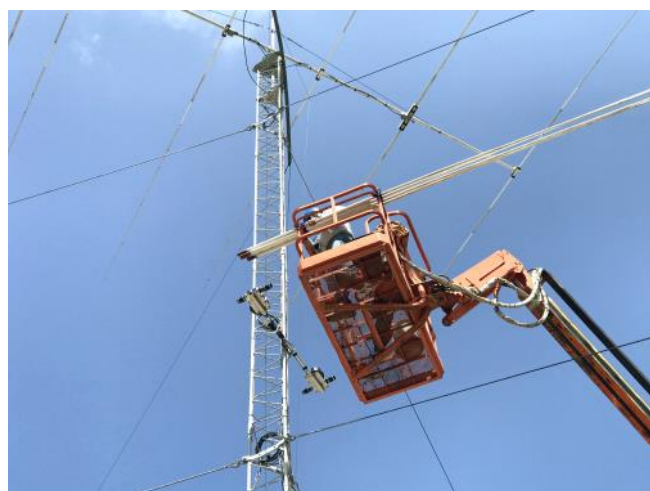
The SteppIR boom installed
