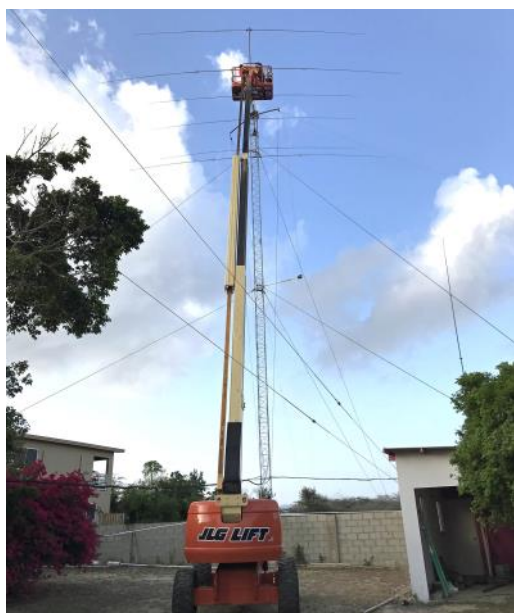
The lift maxed out to reach the 40m driven element
