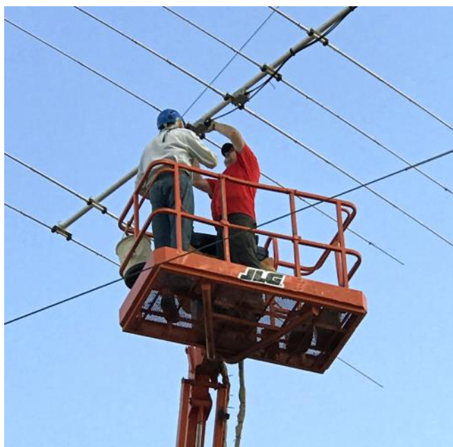
Replacing the 10m loading coil
