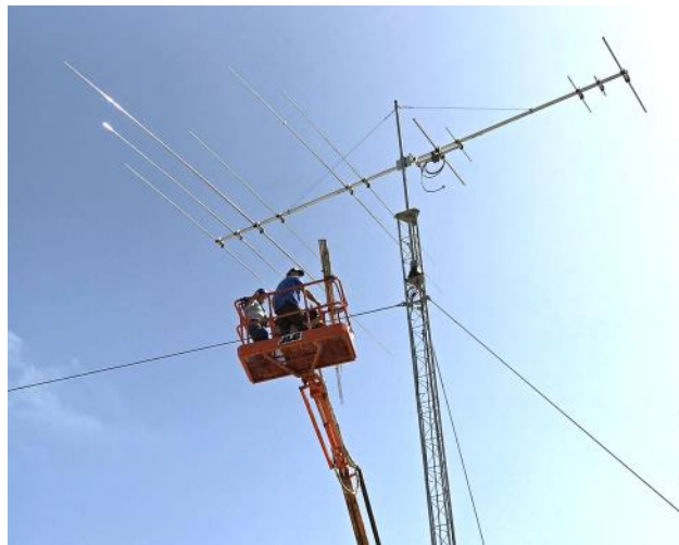
Installing elements on the Mid-Tri
