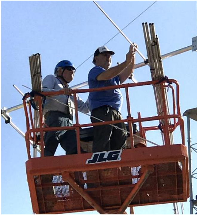
Each half element is held on to the center section by one screw and nut
