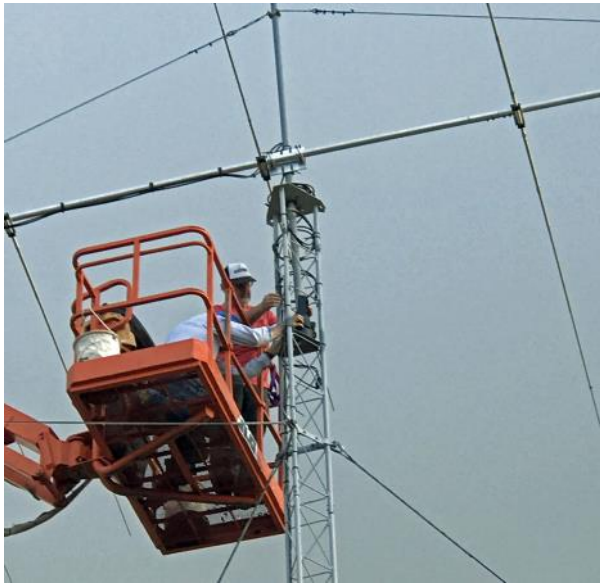
Swapping out the rotor on the 1015
