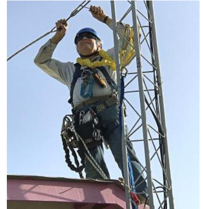
Ed tightening the lower guy, which passes right over the roof of the house
