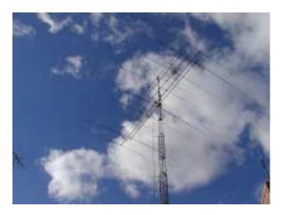
N6TV's antenna system sits on a single 89-foot tower. At the top is an 80 m rotary dipole. At the bottom is a 3-element 40 m yagi. In between, from bottom up, are 5 element monobanders for 20, 15 and 10.
