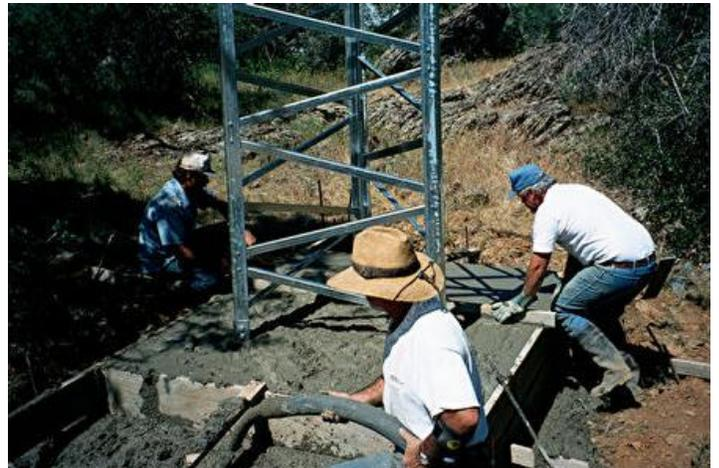
Topping off the tower rebar-ed into the rock. You can see a stream of concrete coming out of the hose.
