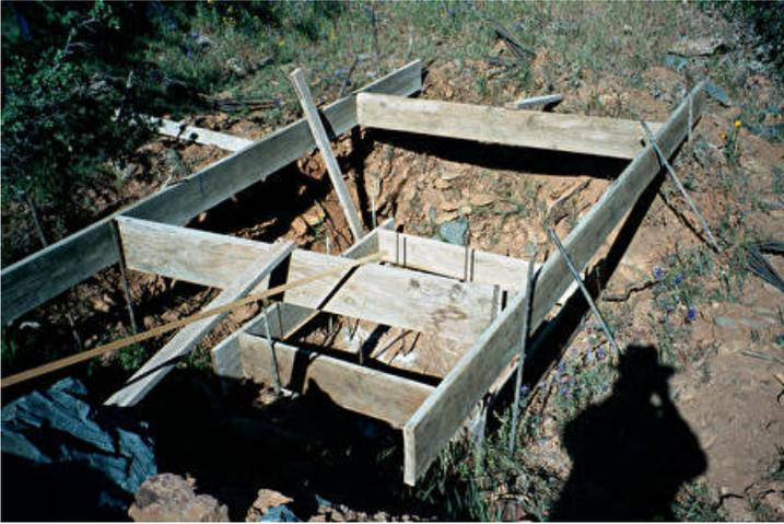
What do you do when the backhoe is half way to spec depth and hits solid rock that, in the opinion of the backhoe operator, “goes half way to China”? The silly thing to do is spend \$1200 blasting it out so that you can fill the hole up again with concrete. But, if you are deep enough to clear the stub legs, you drill into the rock and use rock epoxy to cement in some rebar. The rebar is just visible in this photo, to the left of “the shadow”.
