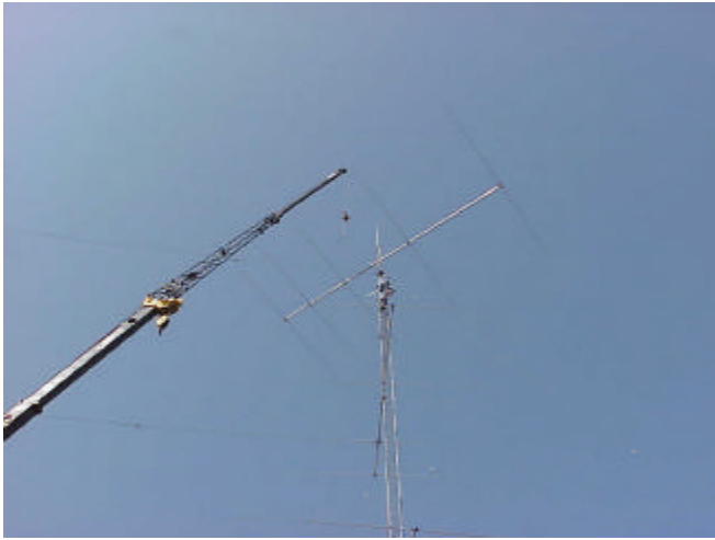
At WC6H, a 5 element KLM 20m Yagi and a 4 element KLM 40m Yagi were taken down to replace a bent mast. The crane is sure a good way to move things around up there!
