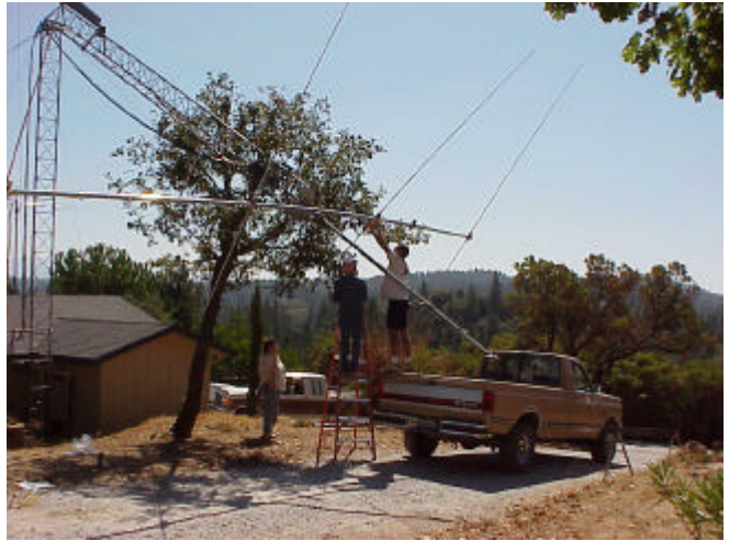
At K6DB/K6KAY a Force-12 5 element 15m Yagi was put up to round out the collection: 80m rotatable dipole, 2 el 40m, 5 el 20m, and 6 element 10m Yagis! (I hope that's a tilt-over tower! If not, Ken and Kay have some more work in store for them!... ed)
