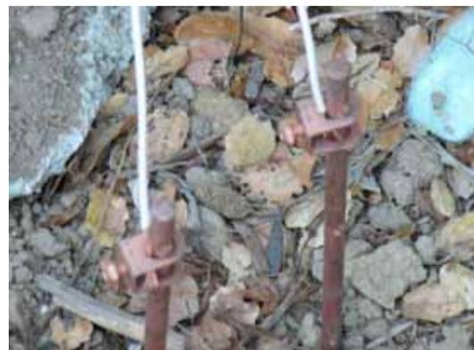
Using Velcro, I mount the two head-end modules on my house's southern fence, drive a pair of ground rods into the ground nearby, and wire each rod to one head-end's ground terminal.
