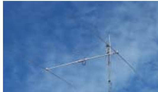
The 40 meter antenna goes up the tram.
